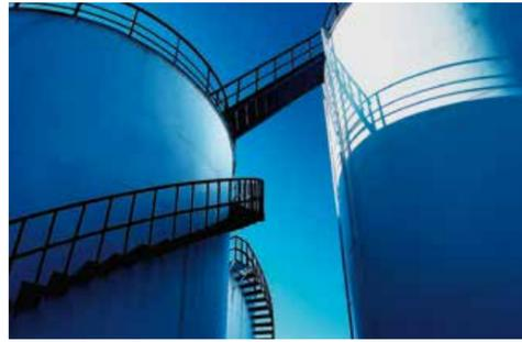
A major United States oil refinery chose our Hempaline Defend 630 Solvent Free Novolac Epoxy Lining as an interior tank lining for a 200 foot / 61 metre diameter sour crude oil storage tank.
