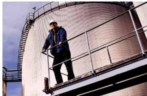
A major US oil company was experiencing corrosion in its sour crude oil tanks. Chemicals and water in the oil were causing severe pitting and corrosion at the bottom of the storage tanks. To combat this, we recommended Hempaline Defend 740 Vinyl Ester Mat Reinforced Lining. The addition of the reinforcement mat not only affords greater barrier properties but contributes to the materials ability to withstand flexure and impact.
